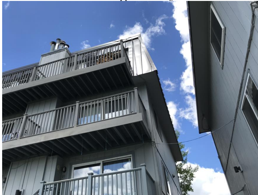
Firewood on upper deck-right side
