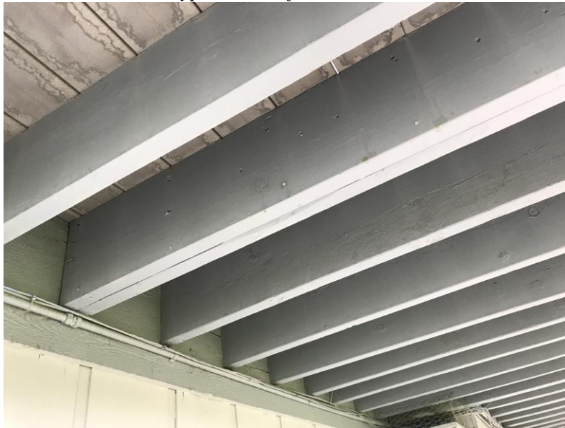
Typical deck joists
